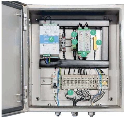
Master unit at the SCADA side
